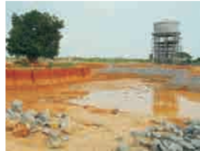
Lake with boating facility-work in progress
