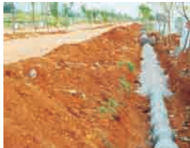
Underground drainage-work in progress
